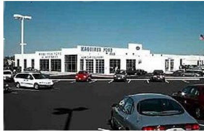
Parking lot lighting
